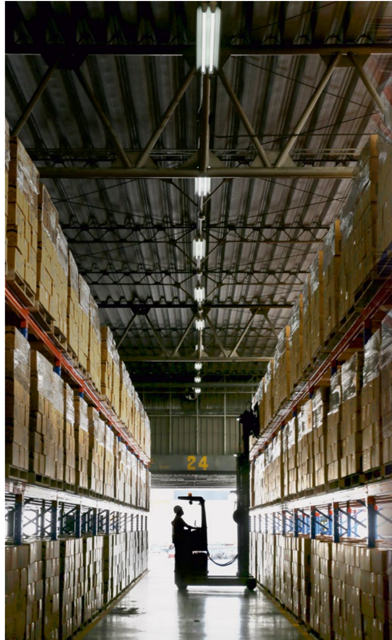
BEFORE lighting modernization
